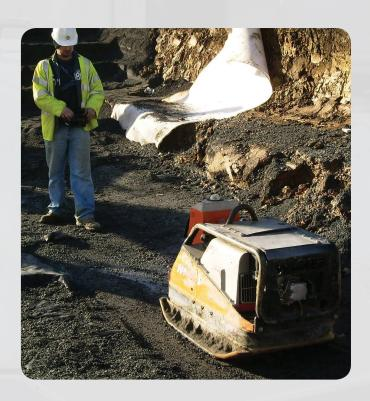
Ergonomic design and remote control operation makes compaction simple and straightforward.
